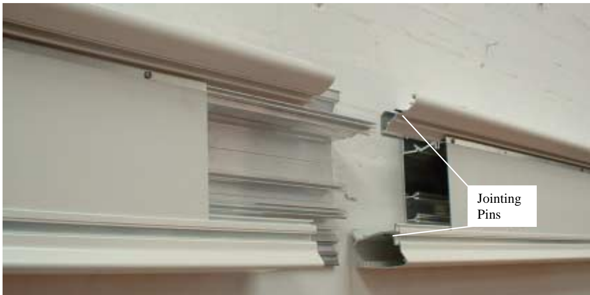
Figure 3 – Preparation for Trunking Joining
