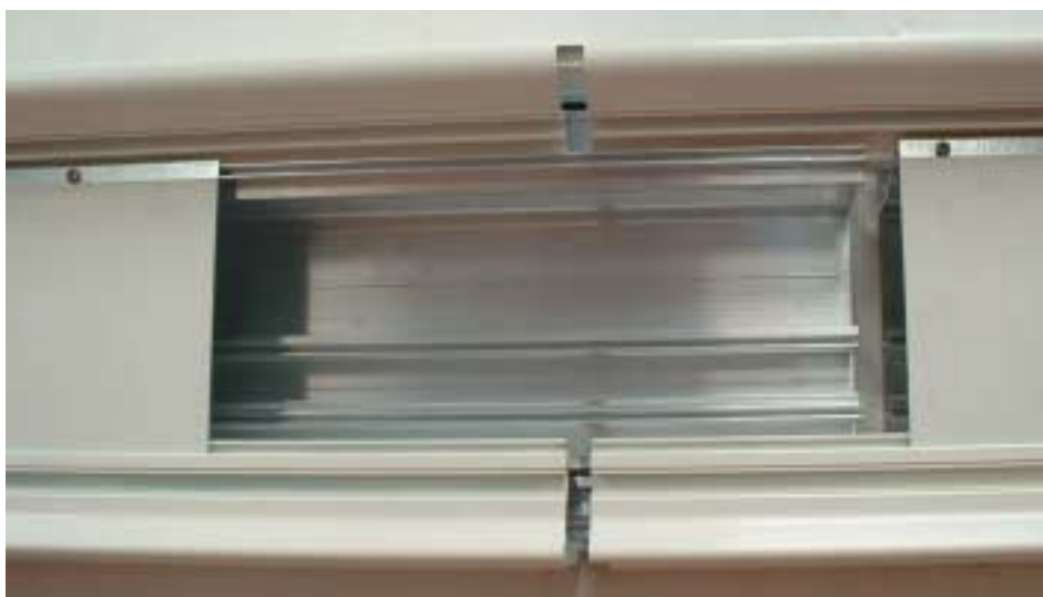
Figure 4 – Trunking Joining
