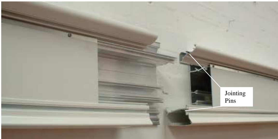
Figure 3 – Preparation for Trunking Joining
